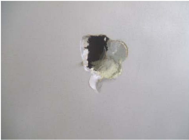
Figure 1. Damaged Gypsum Board
