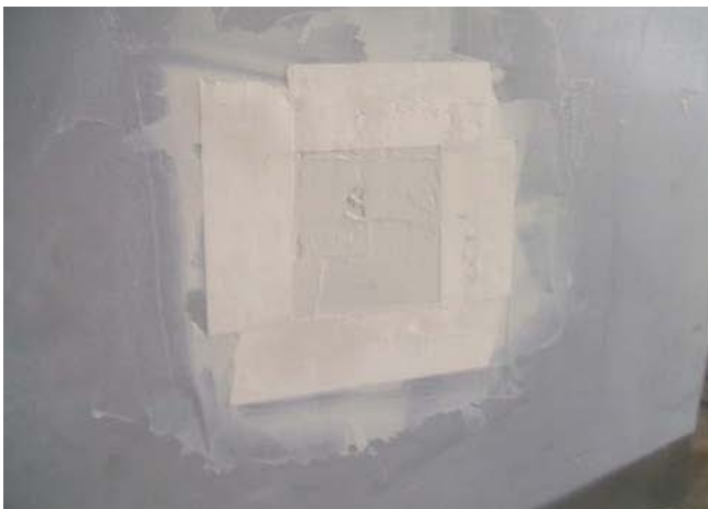
Figure 5. Tape and Finish Patched Area
