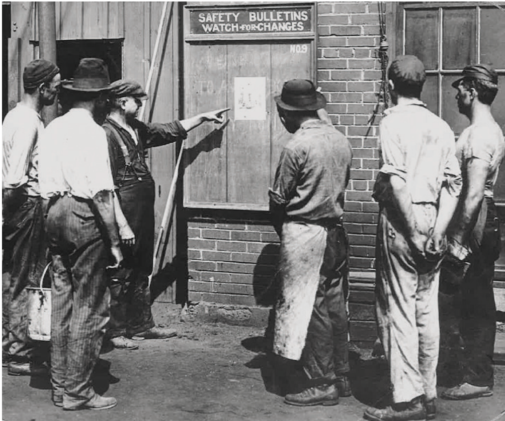
Taken just two years after the Gypsum Association was founded, this 1932 image of an unidentified gypsum manufacturing plant shows early safety-related efforts.
